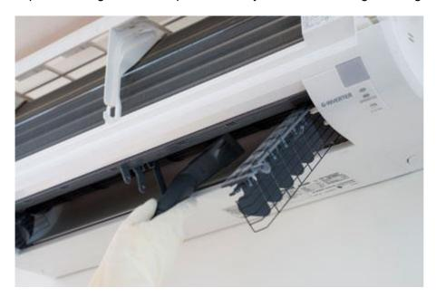
For easy cleaning, the unique Mitsubishi Electric Quick clean design enables removal of the front panel and air flow vents providing open access, including to the fan. Regular cleaning of the indoor unit improves performance, reduces energy consumption and extends the life of your air conditioner. Quick Clean Design is available on these models:
