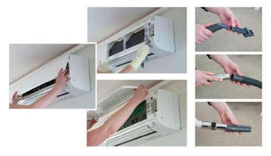
Cleaning your heat pump regularly ensures optimum operation efficiency and reduces unnecessary power consumption. We recommend cleaning your heat pump as often as every two weeks in order to utilise its full performance. To ensure your heat pump works as efficiently as possible use this easy to follow guide along with your Quick Clean Kit.
